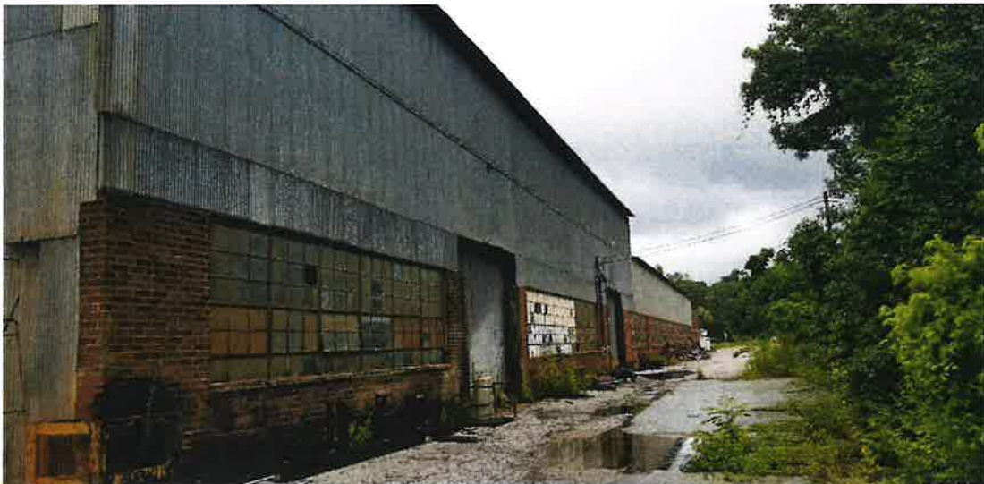
Photograph 2 Maddox Foundry southeast property line
